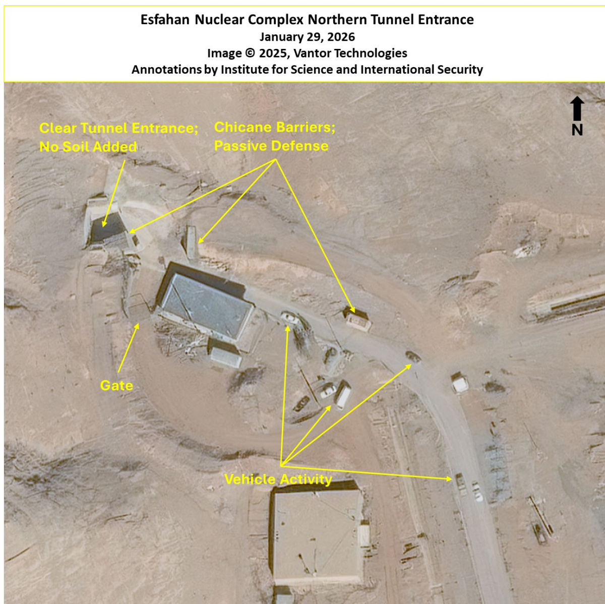
Figure 4. The northernmost tunnel entrance appears to remain open and vehicles are present near the entrance.
